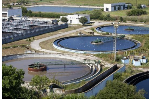
Wastewater plants and sampling
